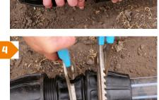
While holding the body tighten the nut all the way to the flange using multi-grips. The fitting is now fully installed.
