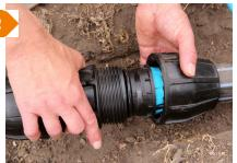
components on to the pipe and bring the body onto the
