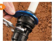
righten nut firmly with a wrench. Nut will not butt against the body flange when the pipe size is at the top end of the fitting tolerance.
