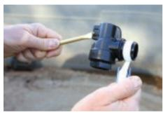
Apply PTFE tape or approved sealant to the thread ensuring sufficient is applied to ensure a watertight seal
