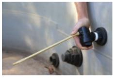
2. Screw into the female thread by hand until firm.
